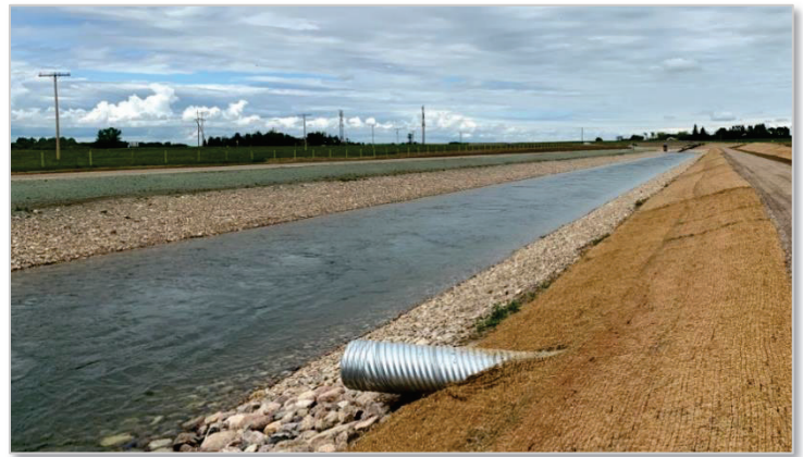
Figure 3: The M1 Canal from Lake Diefenbaker, recently rehabilitated to modern standards (including a lining comprised of rubber and rocks and a reduced slope to enable improved construction access)
