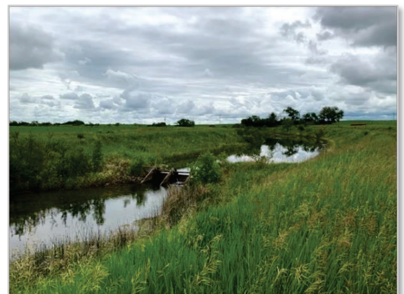
Figure 2: An existing portion of the West Main Canal, showing encroaching vegetation, intense slope, and a lack of lining
